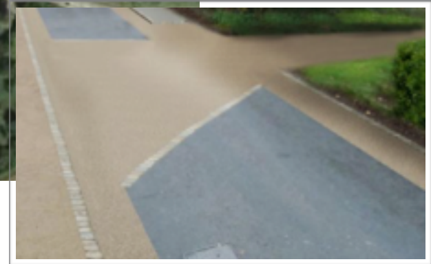
Example of type of road colouring which indicates likely crossing point.
